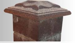
This term refers to the use of "Father's Hat Stone" as a coping element, which is designed to protect the upper part of buildings. This stone is commonly used on the edges of roofs or tops of walls to help direct water away and protect the structure.
